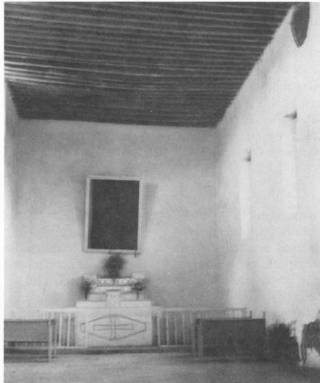
Interior of the presidio church of San Carlos
